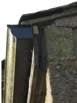
Figure 28 - Open end of fascia at eaves
