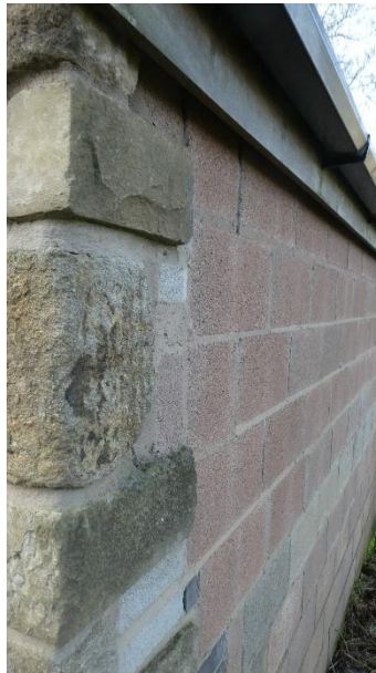
Figure 73 - Exposed blockwork to rear of garage
