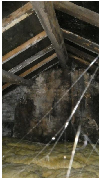
Figure 2 - Party wall/gable wall from within roof void
