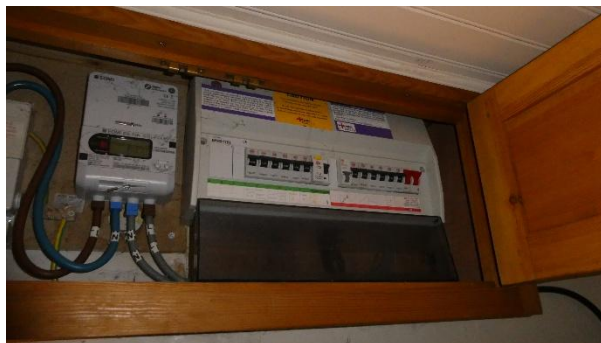
Figure 69 - Consumer unit within main circulation space
