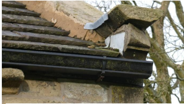
Figure 12 - Stone kneeler to front right roof parapet
