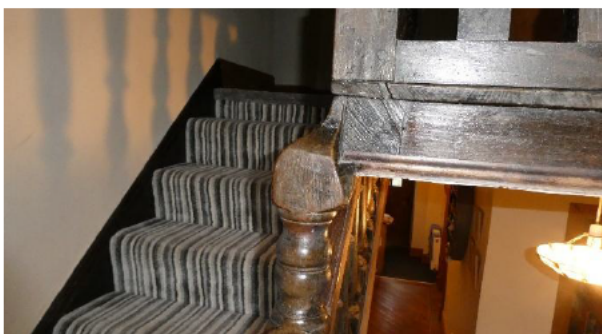
Figure 83 - First floor landing load transferred through newel post of stairs
