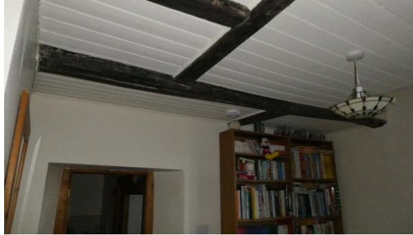
Figure 47 - Historic timber girders to base of stairs
