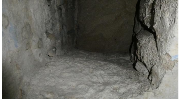
Figure 52 - Flue within cellar capped with stone
