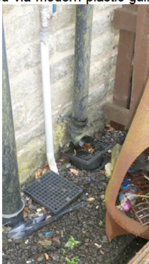
Figure 72 - Raised gullies to rear
