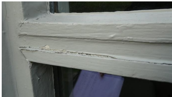
Figure 24 - Peeling painted finish to timber window frames
