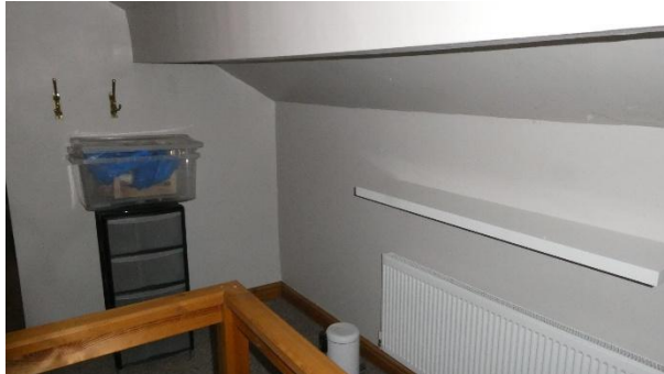
Figure 86 - Lower ceiling within roof void at higher risk of condensation forming
