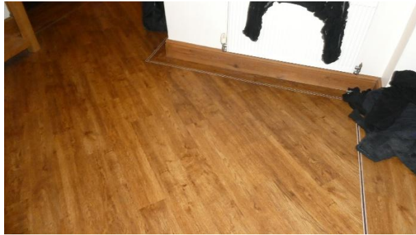
Figure 46 - Bulge in floor of ground floor corridor observed in this area
