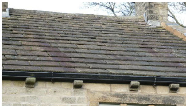
Figure 15 - Aluminium front gutter
