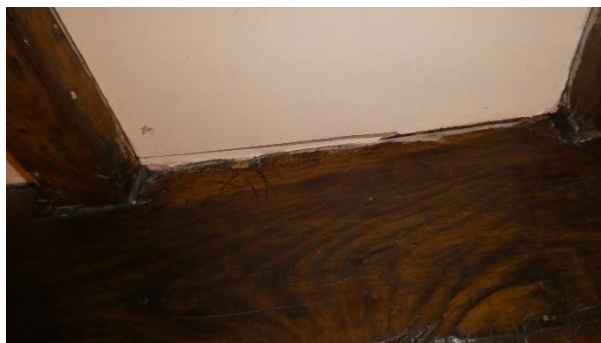
Figure 41 - Cracking between plaster and timber joists
