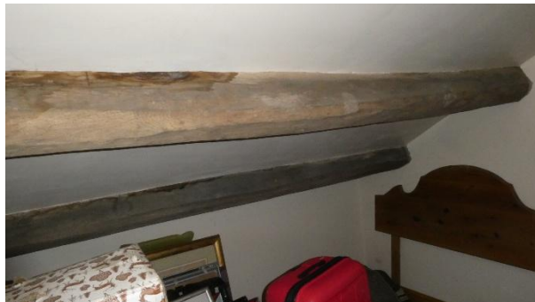
Figure 33 - Timber purlins to Storage area
