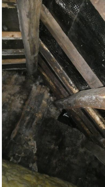
Figure 11 - Visqueen underlay over rafters
