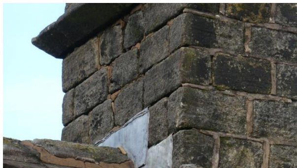
Figure 5 - Weathered mortar to central chimney stack
