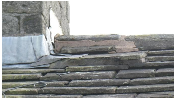
Figure 10 - Mortar fill below slate to rear slope
