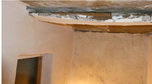
Figure 59 - Rotten timber above stairs to cellar
