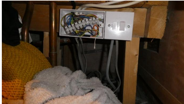
Figure 70 - Exposed wiring to junction box in cylinder cupboard
