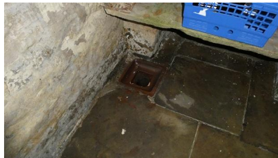
Figure 65 - Drainage gully to floor of cellar
