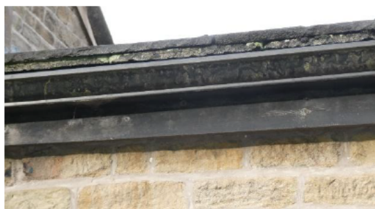
Figure 16 - Aluminium gutters to low level roof
