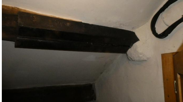
Figure 35 - Steel encasement to rear purlin
