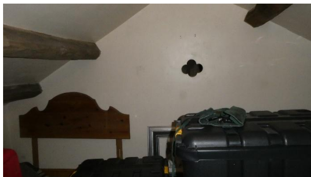
Figure 36 - Hole in stud partition allowing observation into roof void
