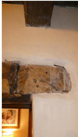
Figure 44 - Cracked and hollow plaster above door of Reception Room
