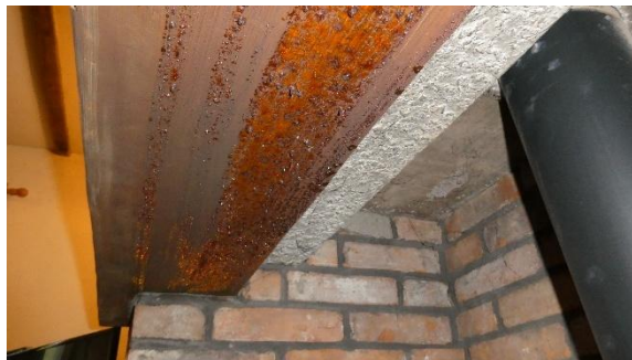
Figure 49 - Heat damage to varnish of mantle
