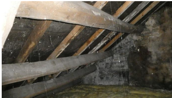
Figure 37 - Purlins below front roof slope
