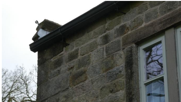
Figure 21 - Open joint in stonework to upper rear corner
