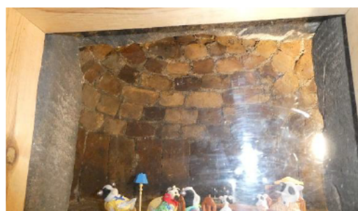
Figure 68 - Historic brick void beneath stairs believed to be an old bread oven
