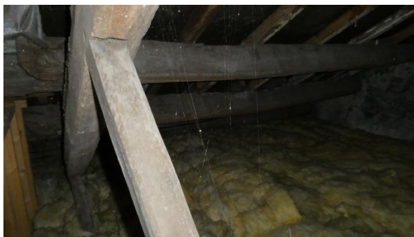
Figure 32 - Purlins supported on timber truss in roof void
