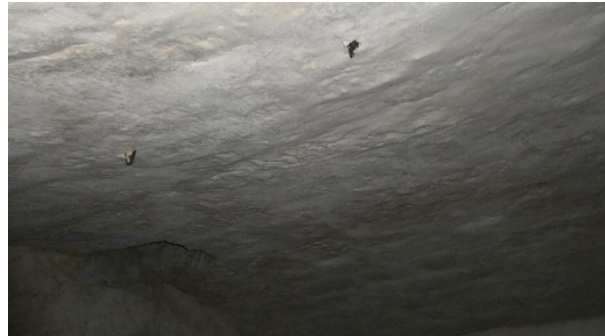
Figure 64 - Corroded fixings to ceiling of cellar
