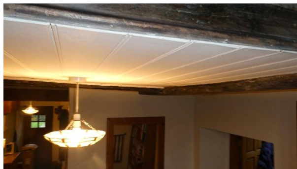
Figure 43 - T&G cladding to ceiling at base of stairs
