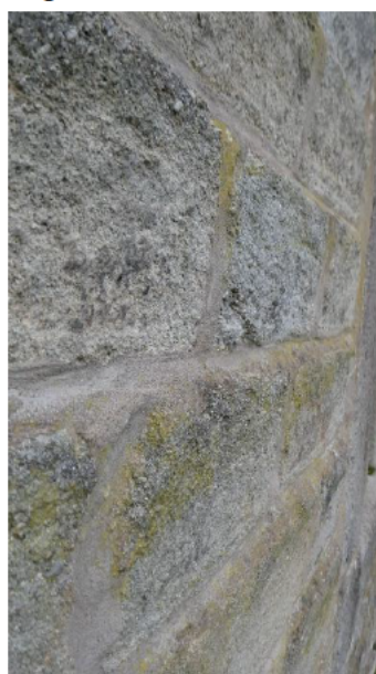
Figure 19 - Water-shot stone finish
