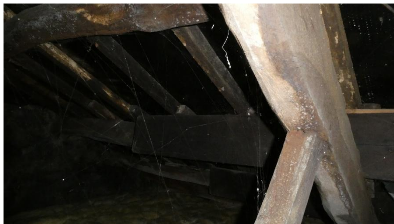
Figure 85 - Mould and condensation seen to roof structure
