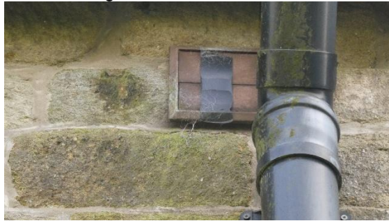
Figure 84 - Taped louvre to bathroom extract fan
