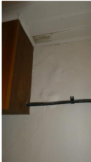
Figure 42 - Damp staining to side of electrical cupboard in main entrance
